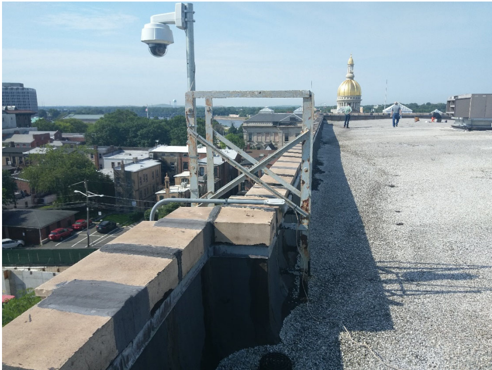
Main Roof Existing Metal Ladder – Looking South
