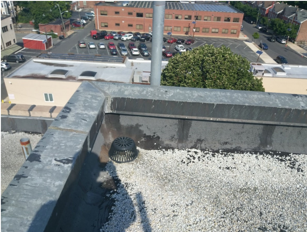
Penthouse Roof – Existing Roof Drain
