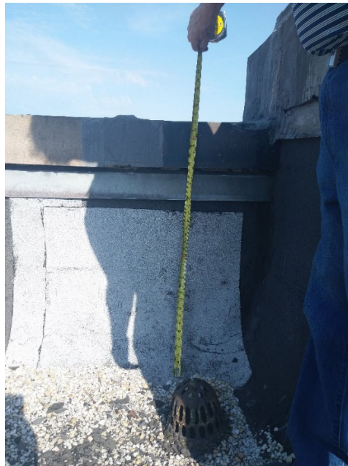
Main Roof – Existing Roof Drain
