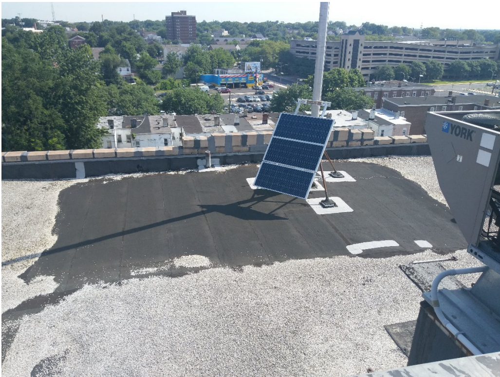
Main Roof – Looking North (Existing Flagpole and Solar Panel)
