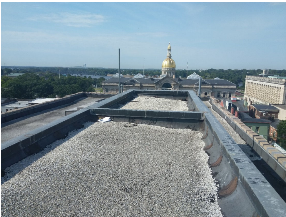
Penthouse Roof – Looking South
