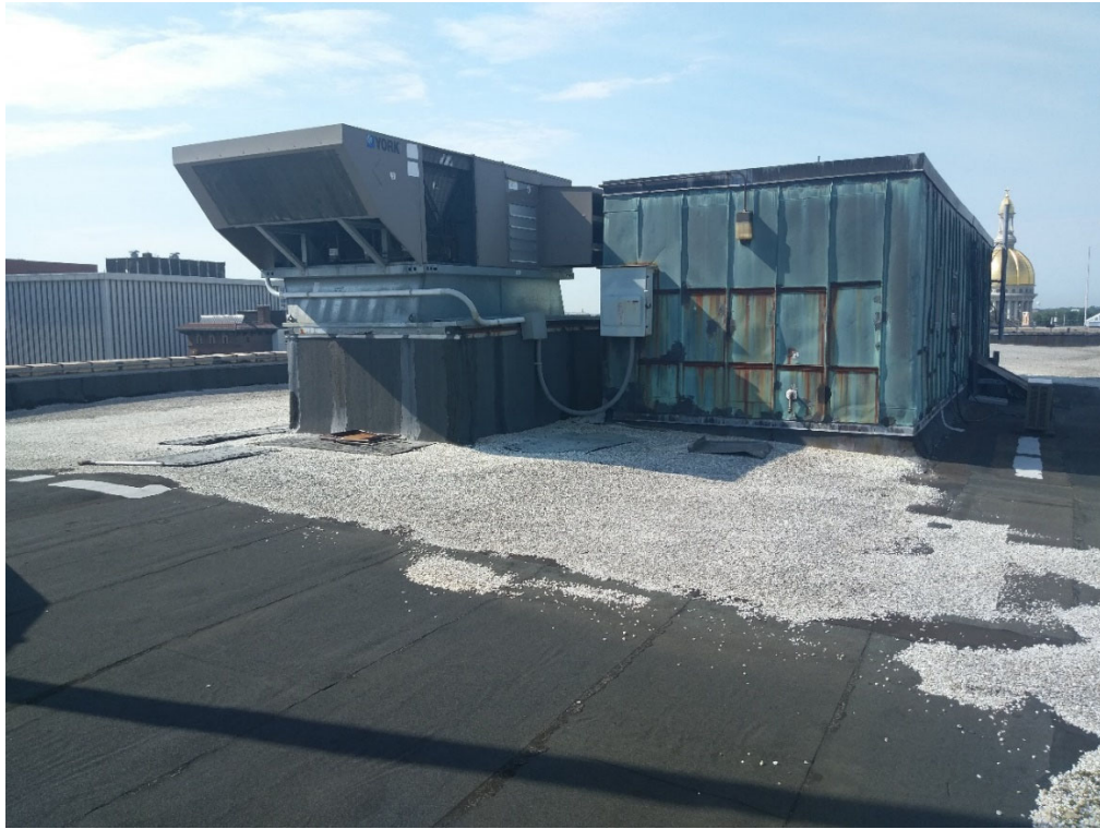
Existing Penthouse Wall and HVAC Unit – Looking South
