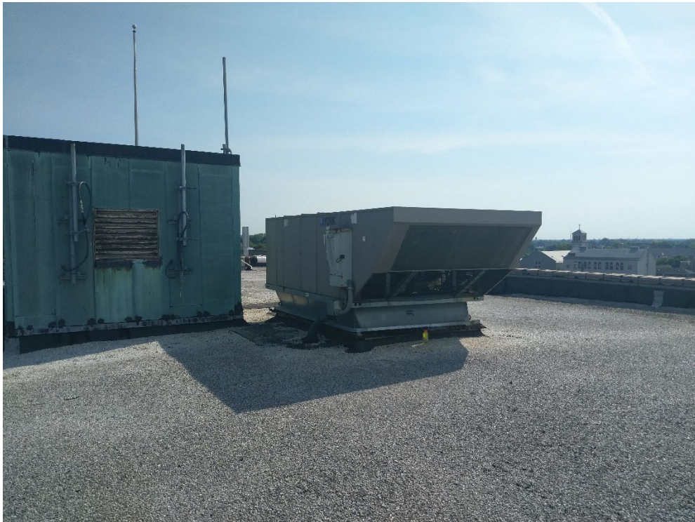
Existing Penthouse Wall and HVAC Unit – Looking North
