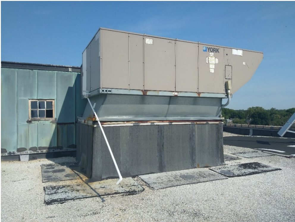
Existing HVAC Unit – Looking North West
