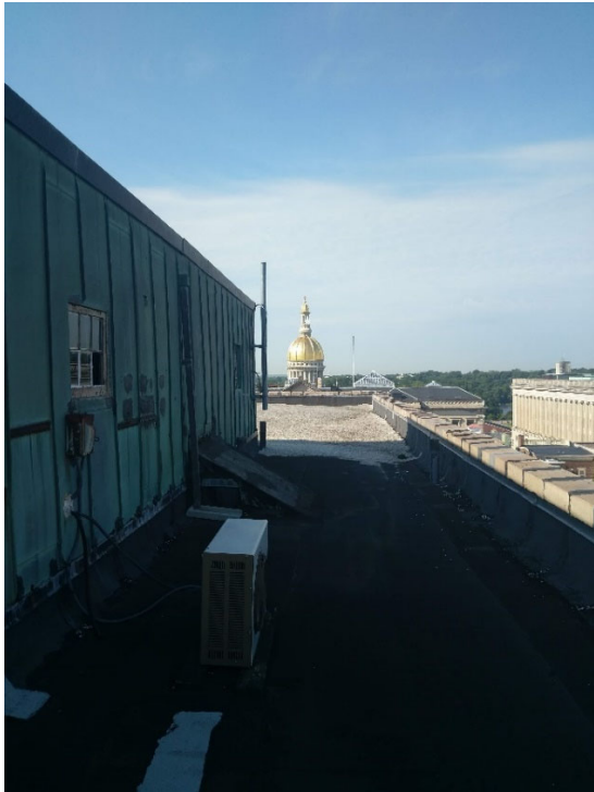
Main Roof – Looking South (Penthouse wall, existing condensing Unit and disconnect switch)
