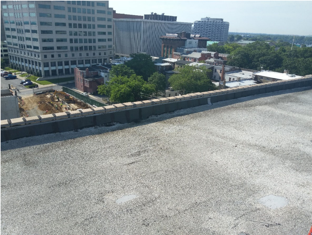
Main Roof – Looking East
