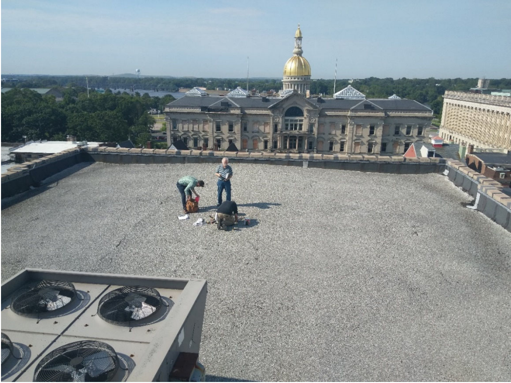
Main Roof – Looking South
