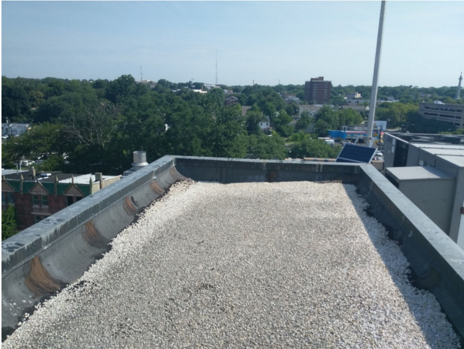
Penthouse Roof – Looking North
