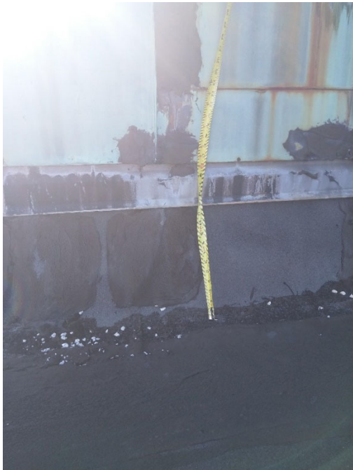
Main Roof – Flashing at Penthouse
