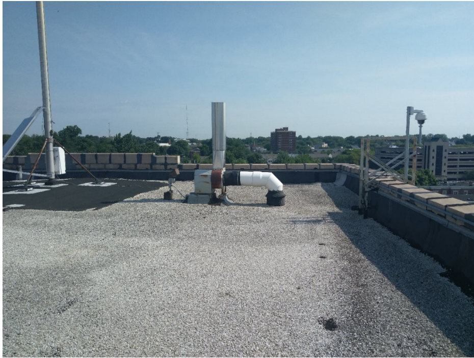
Main Roof Existing Exhaust Duct and Metal Ladder – Looking North
