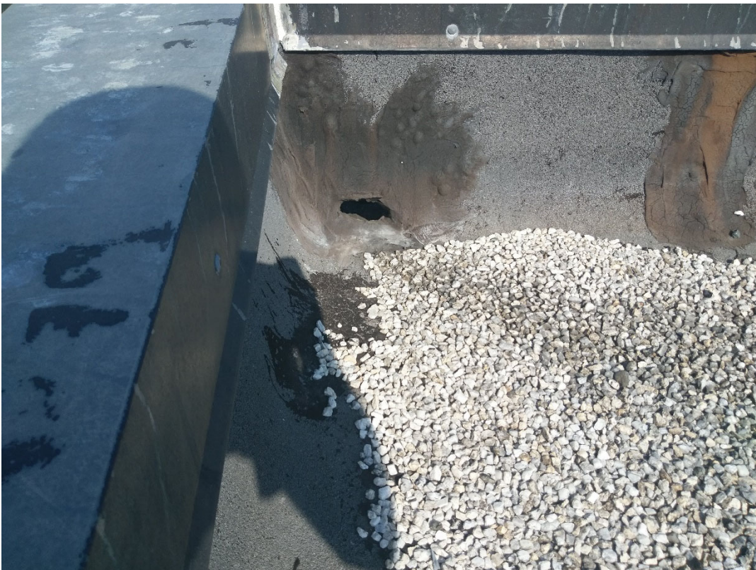
Penthouse Roof – Existing Scupper
