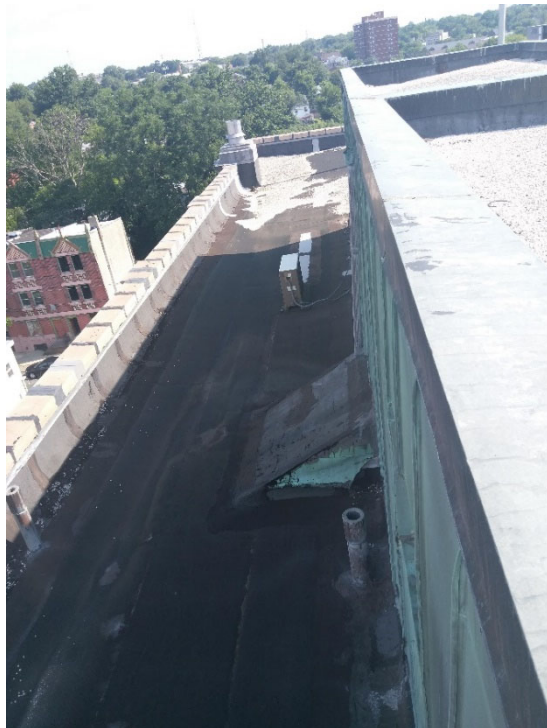
Main Roof – Looking North West (Penthouse wall, existing condensing unit, Stair roof, and vent thru roof)
