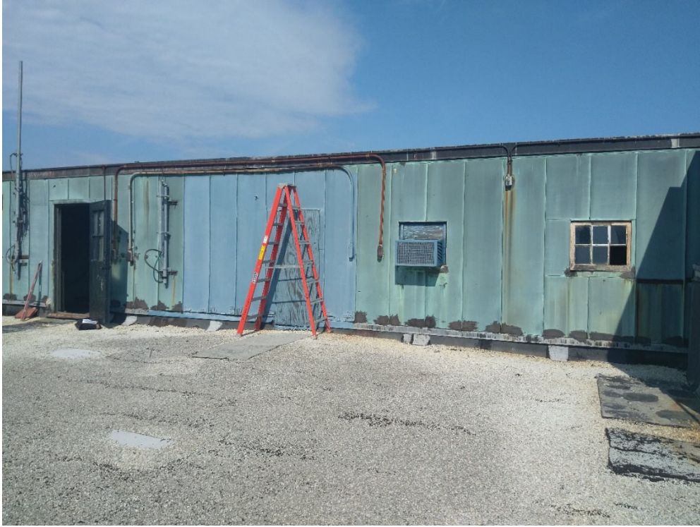
Existing Penthouse – Existing Entry Door
