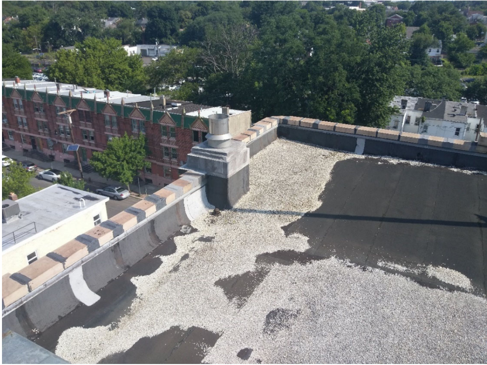
Main Roof – Looking North (Existing Chimney)
