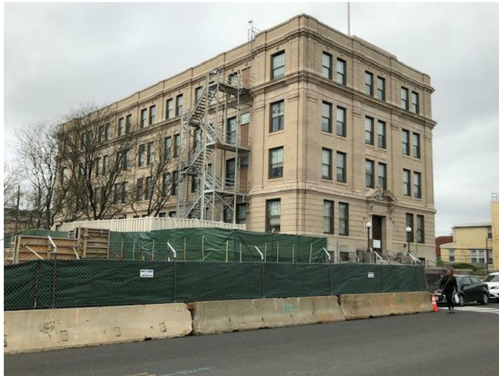
Fire Escape at East Side
