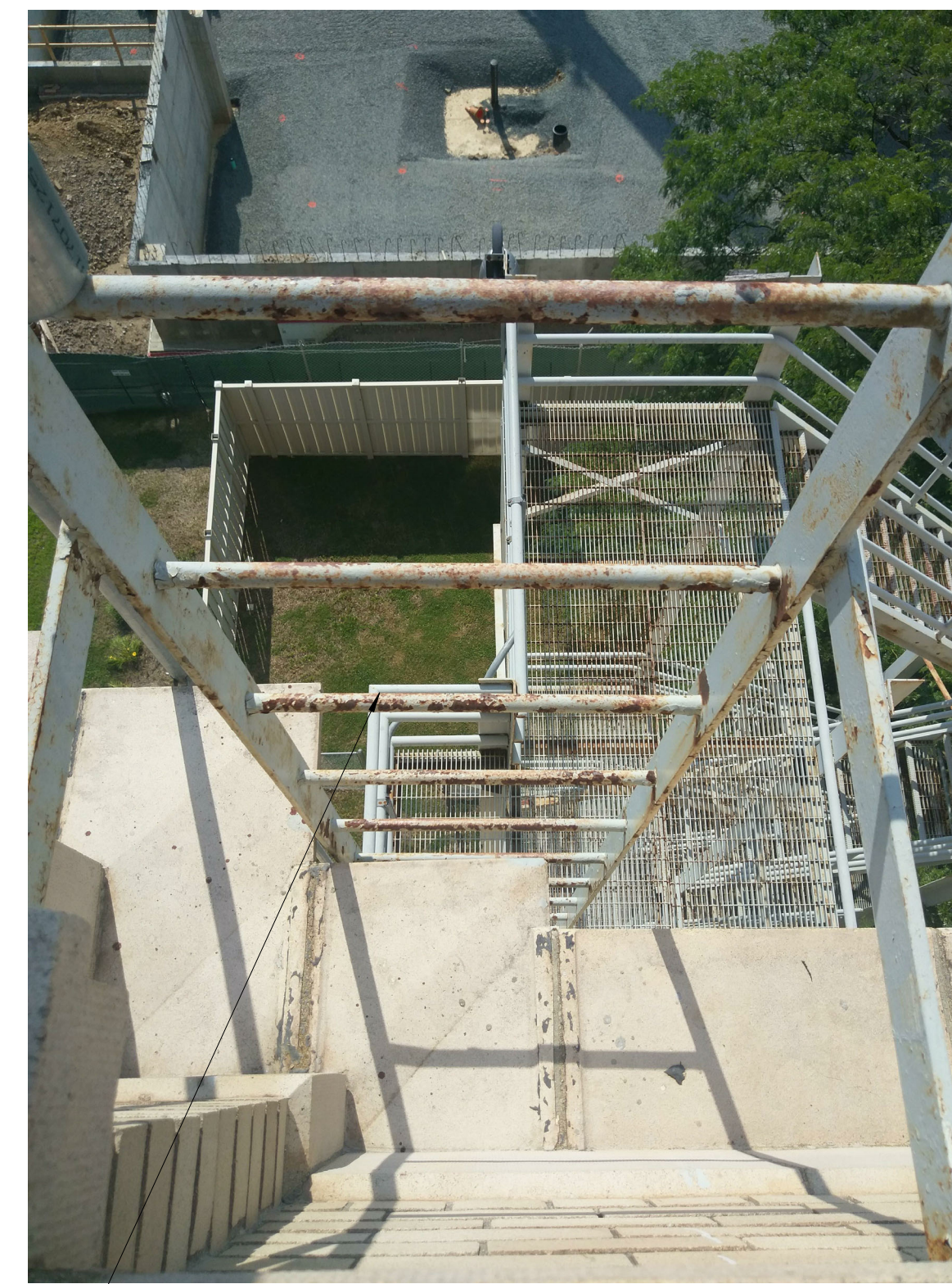
Fire Escape from Roof at East Side
