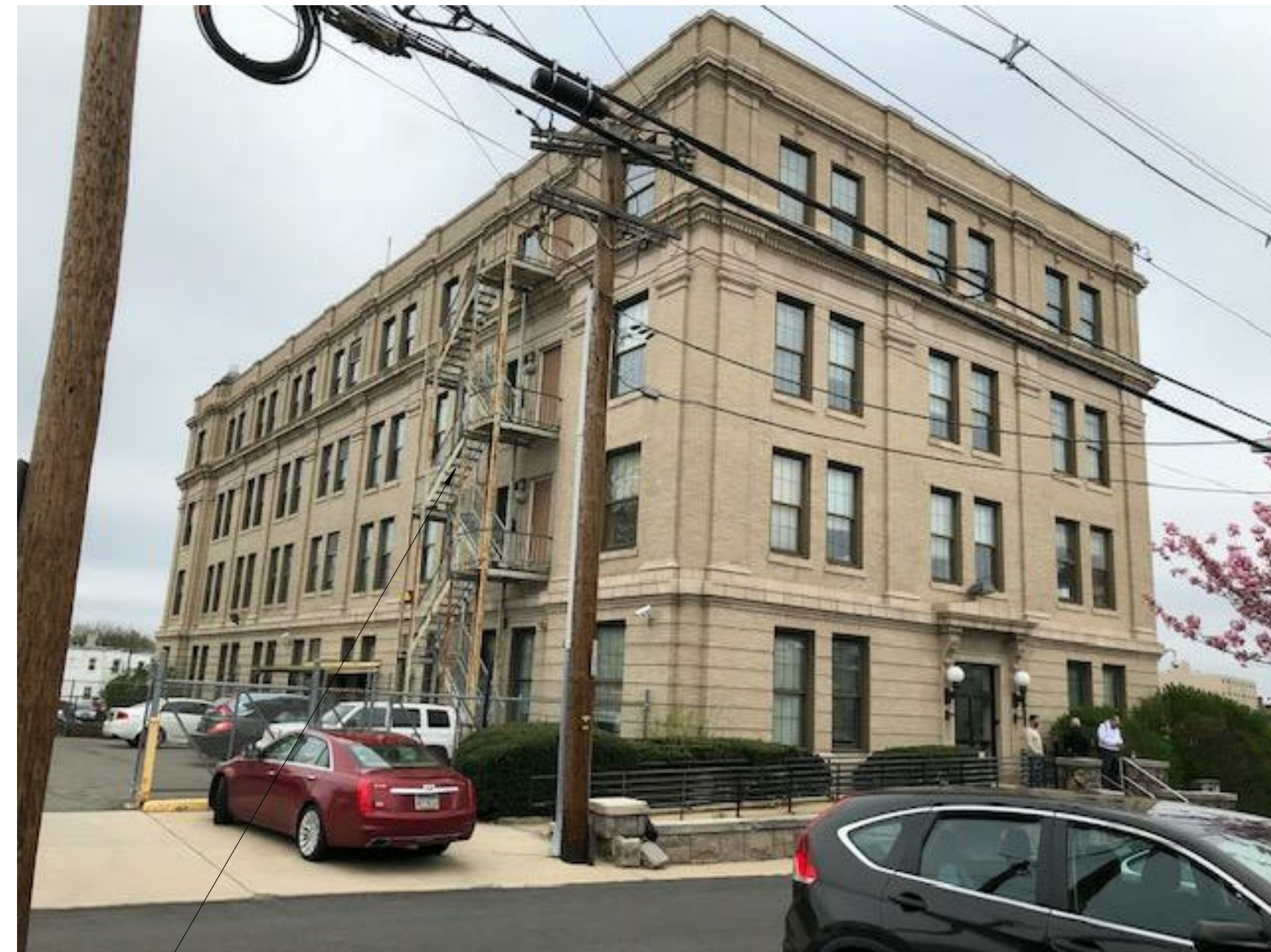
Fire Escape at West Side
