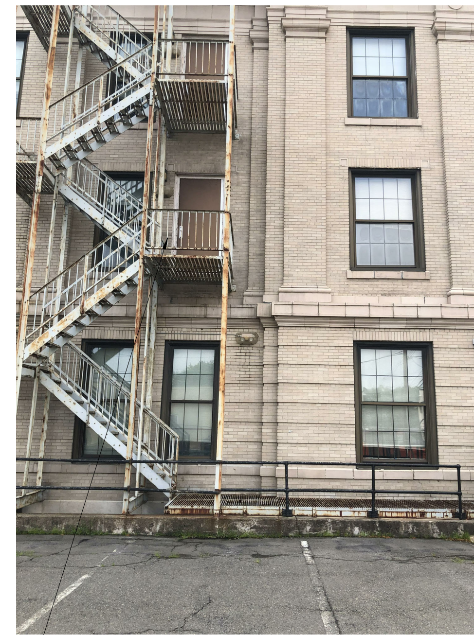
Fire Escape at West Side
