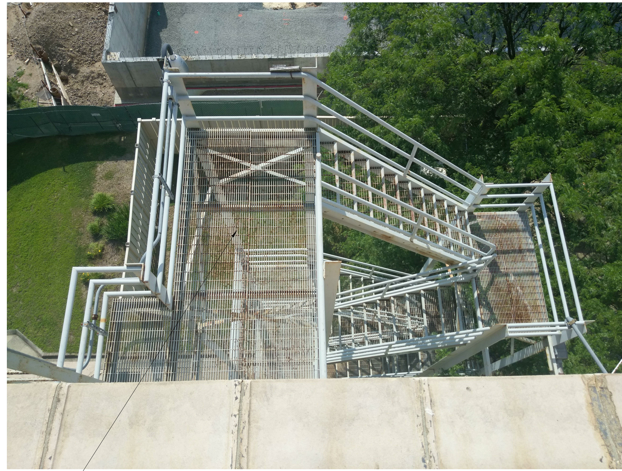
Fire Escape from Roof at East Side
