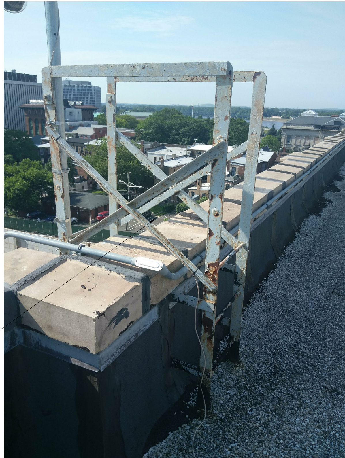
Fire Escape from Roof at East Side
