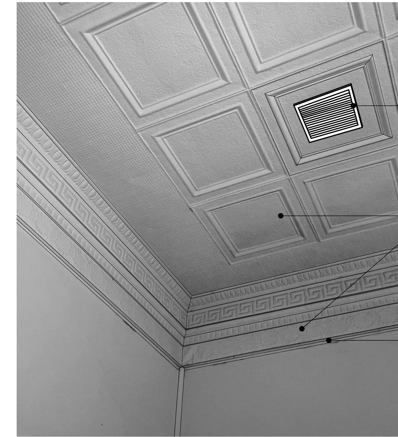
HISTORIC METAL CEILING IN ROOMS 223, 225 AND 226 01
