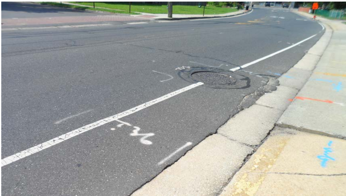
Figure 2. Main utilities marked along the street-side (west side) of the fire station .
