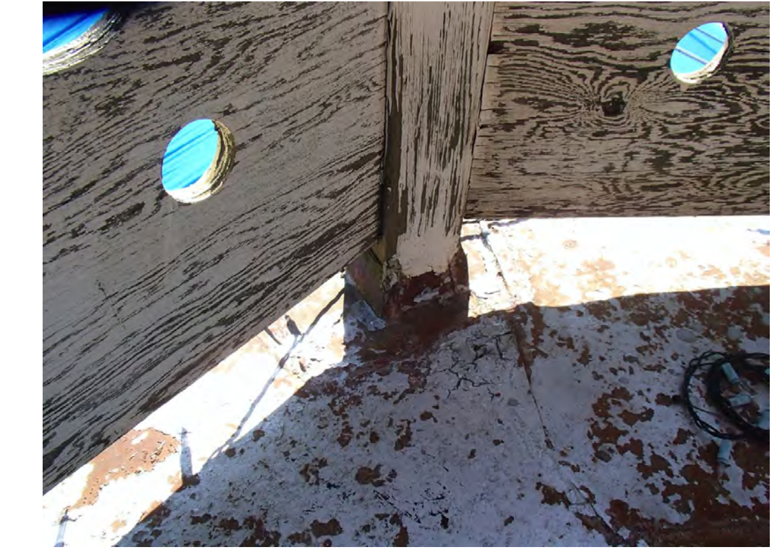
POST AND RAIL RESTORATION (ALT-BID 07) FOLLOW NOTE 1 ABOVE
