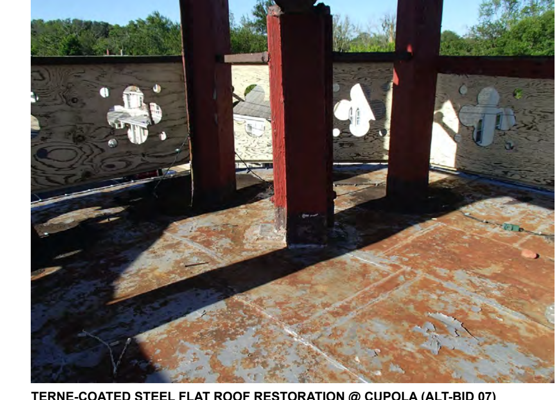
TERNE-COATED STEEL FLAT ROOF RESTORATION @ CUPOLA (ALT-BID 07)
