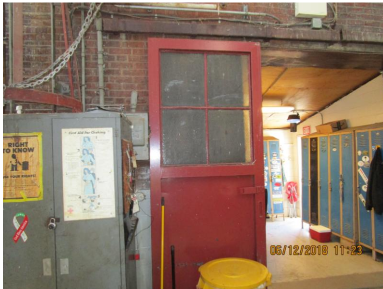
Photograph 12 – Red Paint on Fire Door (LBP)
