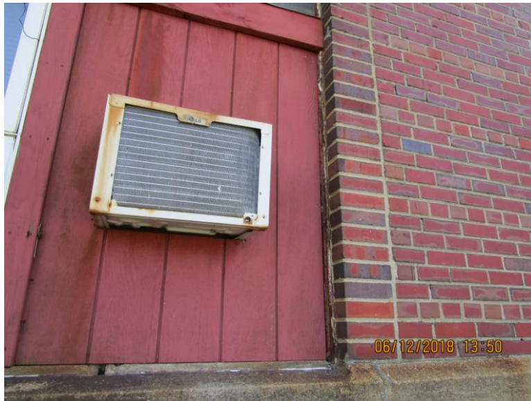
Photograph 5 –Window Caulk (Non-ACM) (No PCB’s)
