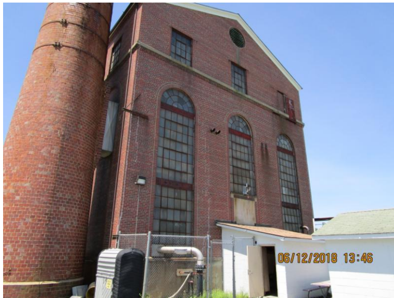
Photograph 6 – Tan Door to Locker Room ( LBP)
