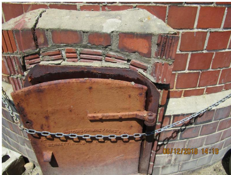
Photograph 4 – Clean out at Base of Stack (Non-ACM)
