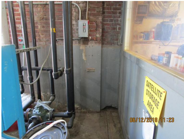
Photograph 11 – Gray Paint on Concrete Walls (LBP)
