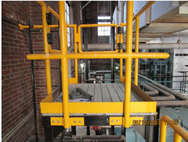
Photograph 14 – Bird feces on building components throughout.
