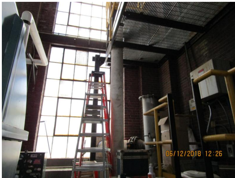
Photograph 10 – Calcium Silicate Pipe Insulation (Non-ACM)
