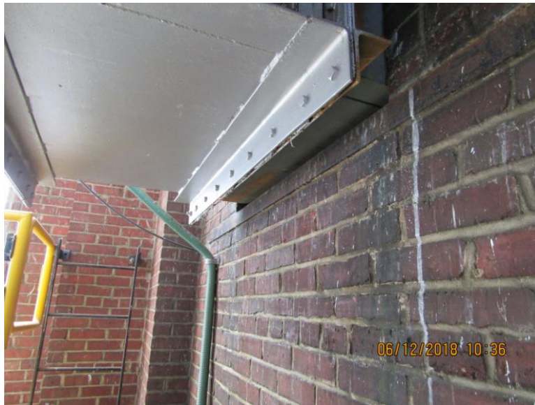
Photograph 8 – Boiler Breaching Seam Gasket (ACM)
