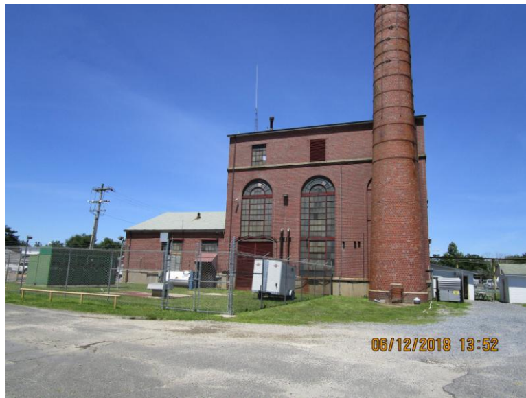
Photograph 2 – Powerhouse Exterior Caulk associated with Stack Bands (ACM)
