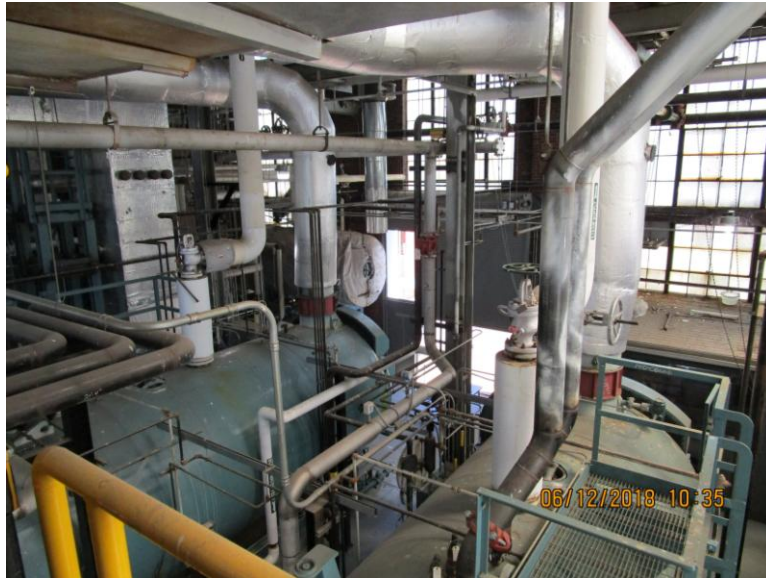
Photograph 7 – Boiler Room Interior General View
