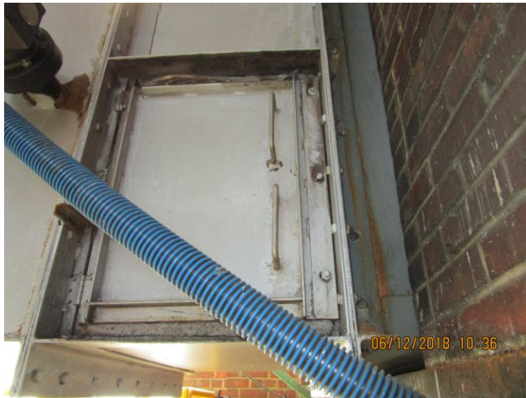
Photograph 9 – Boiler Breaching Door Gasket (ACM)
