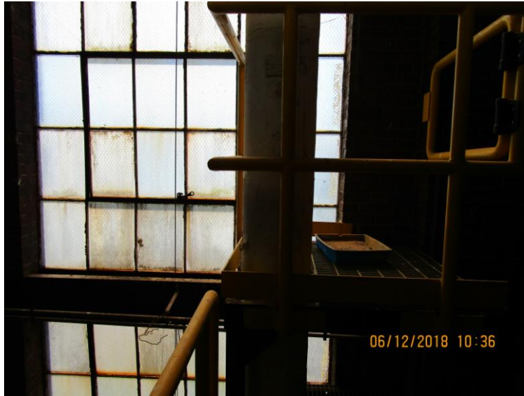
Photograph 13 – Window Mullions (LBP)
