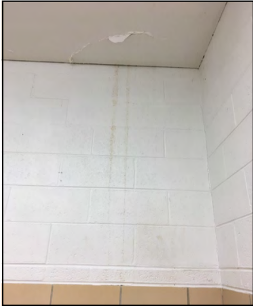
Water Stains from Ceiling in Men's Bathroom
