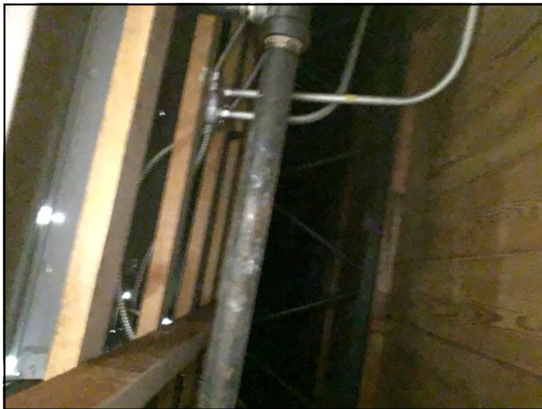
Bare Pipe Above Ceiling - Adjacent Office
