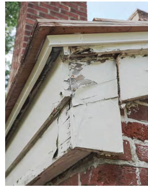
D WOOD REPAIRS REPAIR CORNICE AND FASCIA BOARDS AT CORNER RETURN.
