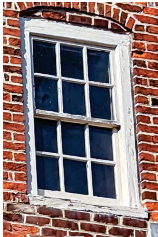
F WINDOW W7 EPOXY REPAIR SHOW SILL.
