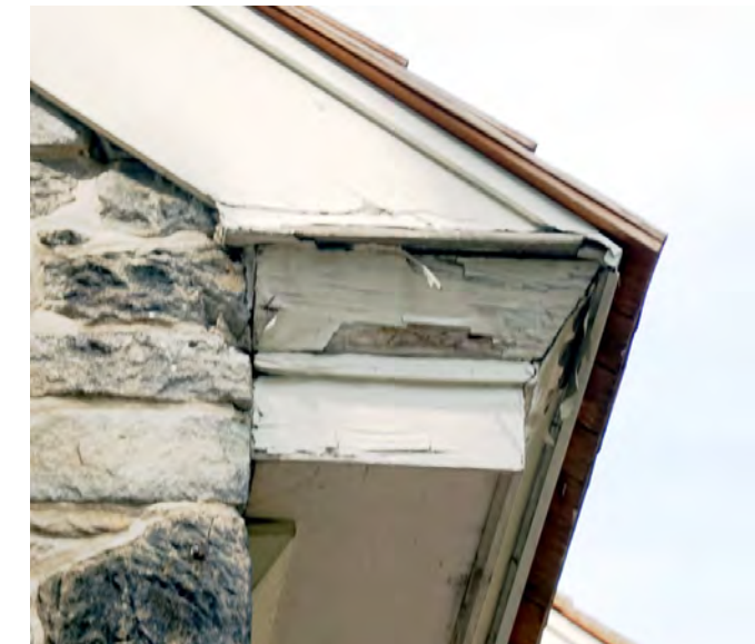
B WOOD REPAIRS @ CORNICE REPAIR CORNICE RETURN
