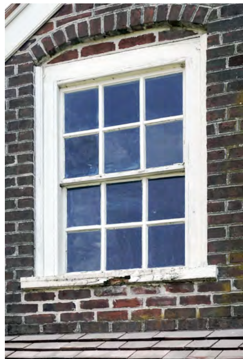
H WINDOW W6 EPOXY REPAIR SHOW SILL.
