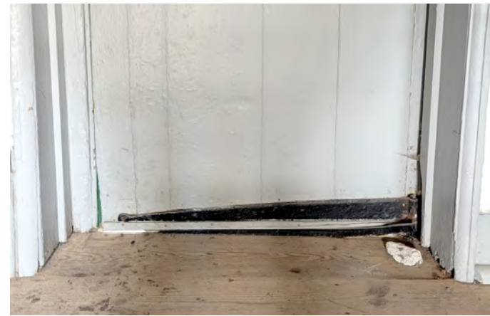
G DOOR D4 REPAIR FRAME, REHANG DOOR, PATCH MORTAR, CAULK JAMBS & HEAD. INSTALL NEW SILL WEATHERSTRIPPING.
