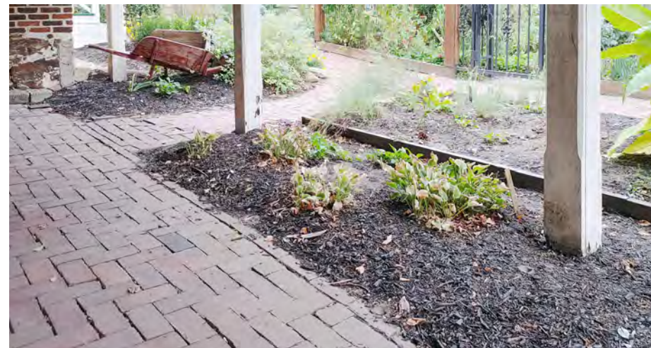
B WOOD REPAIRS @ POSTS REPAIR/REPLACE WOOD POST BOARDS. REGRADE AT BASE TO MINIMIZE POTENTIAL FOR FUTURE DAMAGE. (4 POSTS TYP.)
