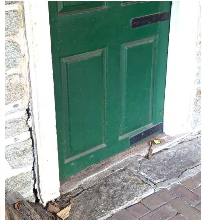
G DOOR D4 REPAIR FRAME, REHANG DOOR, PATCH MORTAR, CAULK JAMBS & HEAD. INSTALL NEW SILL WEATHERSTRIPPING.
