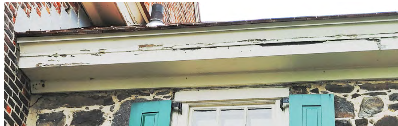
G WOOD REPAIR EXAMPLES OF TYPICAL CONDITIONS IN NEED OF REPAIRS @ CORNICE, FASCIA, RAKE BOARD & MOLDING - SEE ELEVATION PHOTOS FOR SPECIFIC LOCATIONS.
