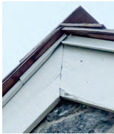
G WOOD REPAIR EXAMPLES OF TYPICAL CONDITIONS IN NEED OF REPAIRS @ CORNICE, FASCIA, RAKE BOARD & MOLDING - SEE ELEVATION PHOTOS FOR SPECIFIC LOCATIONS.
