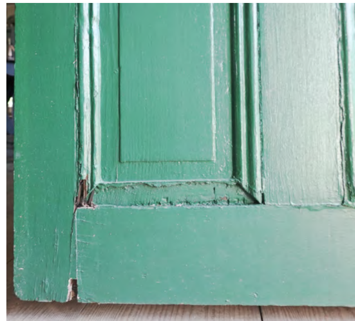
C EXTERIOR VIEW OF DOOR
