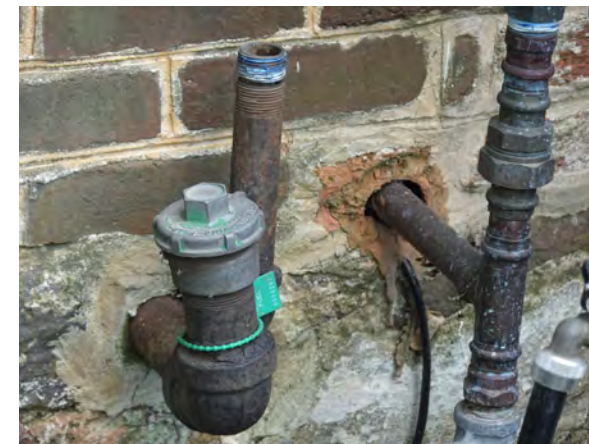
A WALL PENETRATIONS CAULK ALL OPEN WALL PENETRATIONS. REPLACE PREVIOUS CAULK/PATCHING MATERIAL WHERE DETERIORATED, LOOSE OR DISCOLORED..
