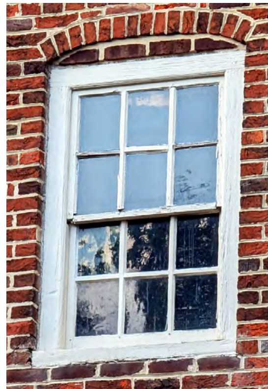
G WINDOW W8 REPAIR & REGLAZE UPPER SASH.
