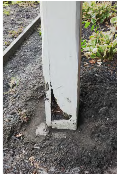
B WOOD REPAIRS @ POSTS REPAIR/REPLACE WOOD POST BOARDS. REGRADE AT BASE TO MINIMIZE POTENTIAL FOR FUTURE DAMAGE. (4 POSTS TYP.)
