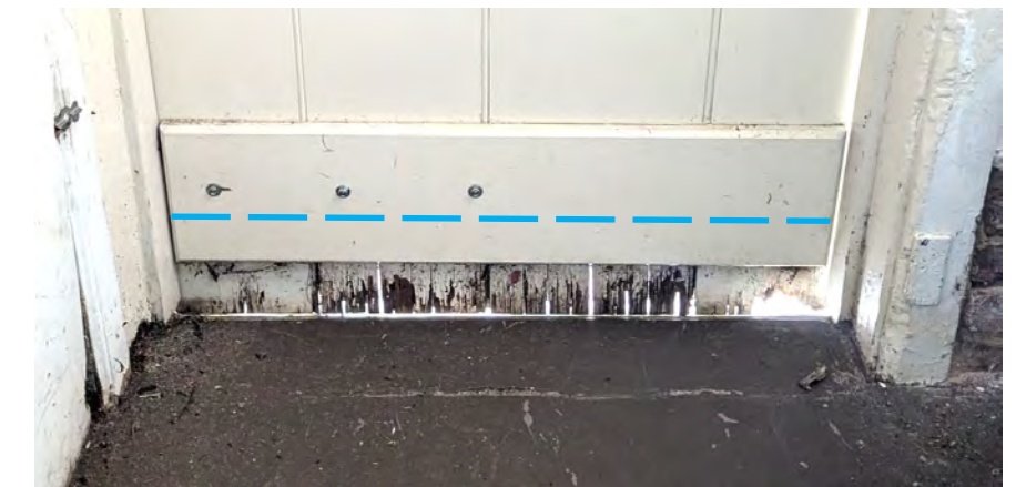
B INTERIOR BOTTOM OF DOOR
