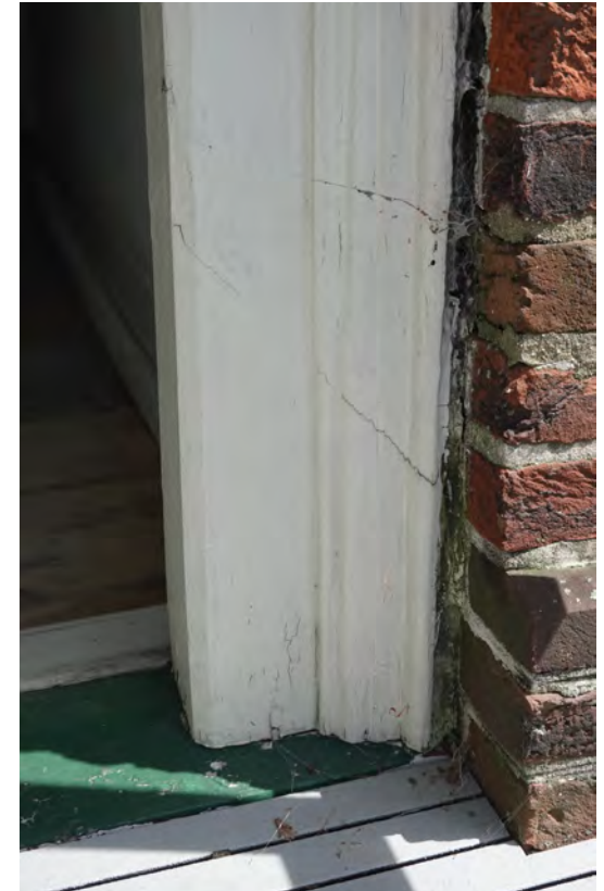
A EXTERIOR VIEW OF JAMB
