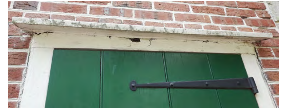
C EXTERIOR DOOR HEAD REPAIR DOOR HEAD TRIM.
