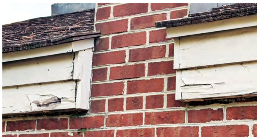
F WOOD REPAIRS REPAIR CORNICE FASCIA & MOLDING.
