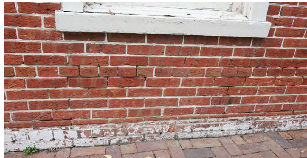
A BRICK REPAIRS, TYP. REPRESENTATIVE VIEWS SHOWING EXAMPLES OF OPEN BRICK JOINTS IN NEED OF REPOINTING. SEE ELEVATIONS FOR DOCUMENTATION OF LOCATIONS.
