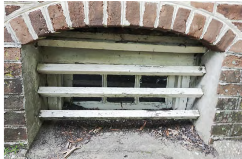
D WOOD REPAIRS EPOXY CONSOLIDATE LOWER BAR AT BASEMENT WINDOW.
