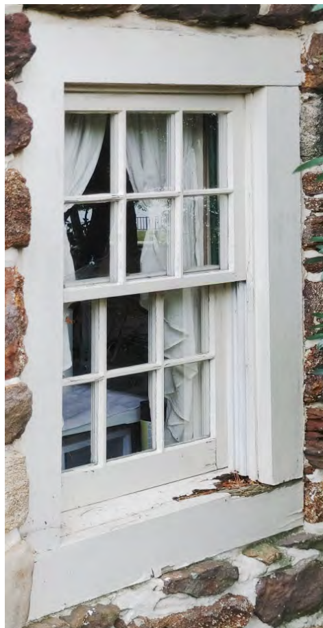
A PHOTO OF EXISTING WINDOW TO BE REPLACED
