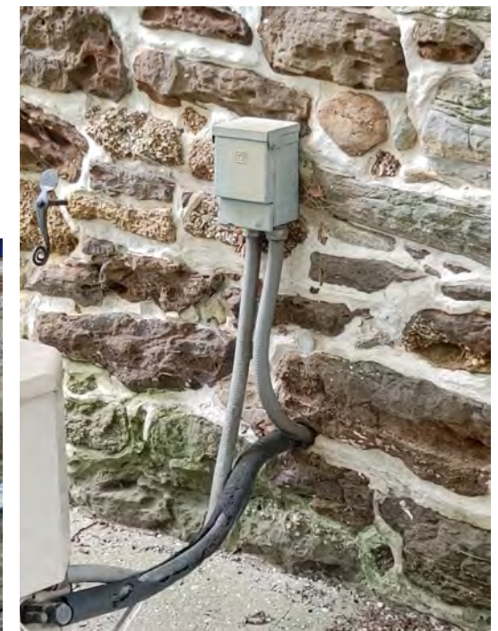
A WALL PENETRATIONS CAULK ALL OPEN WALL PENETRATIONS. REPLACE PREVIOUS CAULK/PATCHING MATERIAL WHERE DETERIORATED, LOOSE OR DISCOLORED..
