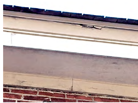
G WOOD REPAIR EXAMPLES OF TYPICAL CONDITIONS IN NEED OF REPAIRS @ CORNICE, FASCIA, RAKE BOARD & MOLDING - SEE ELEVATION PHOTOS FOR SPECIFIC LOCATIONS.
