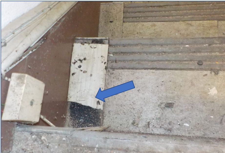
Photograph 3 – Asbestos Containing 9"x9" Grey Vinyl Floor Tile and Mastic
