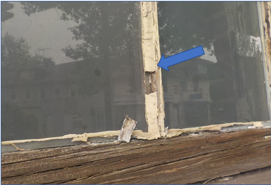
Photograph 5 – Asbestos Containing Window Glazing
