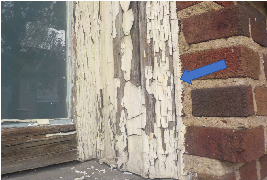
Photograph 6 – Asbestos Containing Masonry Caulk
