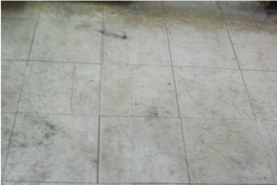
Photograph 7– Asbestos Containing 12”x12” Grey Vinyl Floor Tile and Black Mastic
