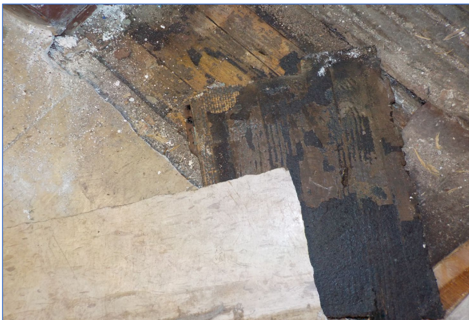
Photograph 2 –Asbestos Containing Multi-Layered Vinyl Floor Tile and Mastic
